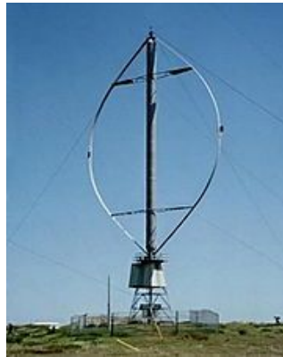
Figure 2.4: 30 m Darrieus wind turbine in the Magdalen Islands "Eggbeater" turbines.
