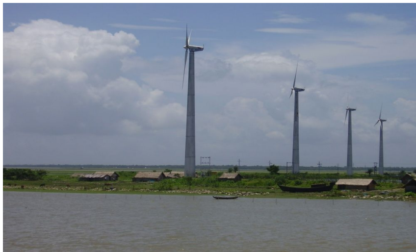
Figure 7.12: Pilot project of 0.90 MW capacity of the Grid Connected Wind turbines in the Muhuri Dam areas at Feni District
