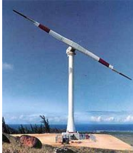
Figure 3.4: The 98 meter diameter, two-bladed NASA/DOE Mod-5B wind turbine was the largest operating wind turbine in the world in the early 1990s
