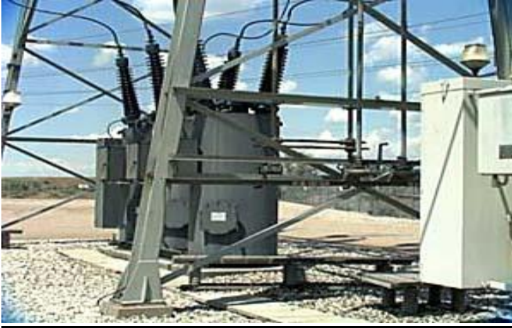
Fig: Oil circuit breakers in a distribution circuit
