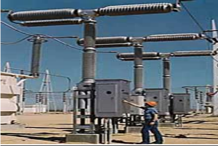
Fig: SF 6 gas power circuit breaker
