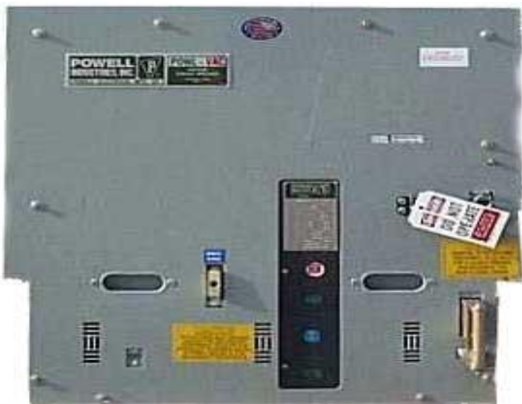
Fig: Vacuum circuit breaker, outside
