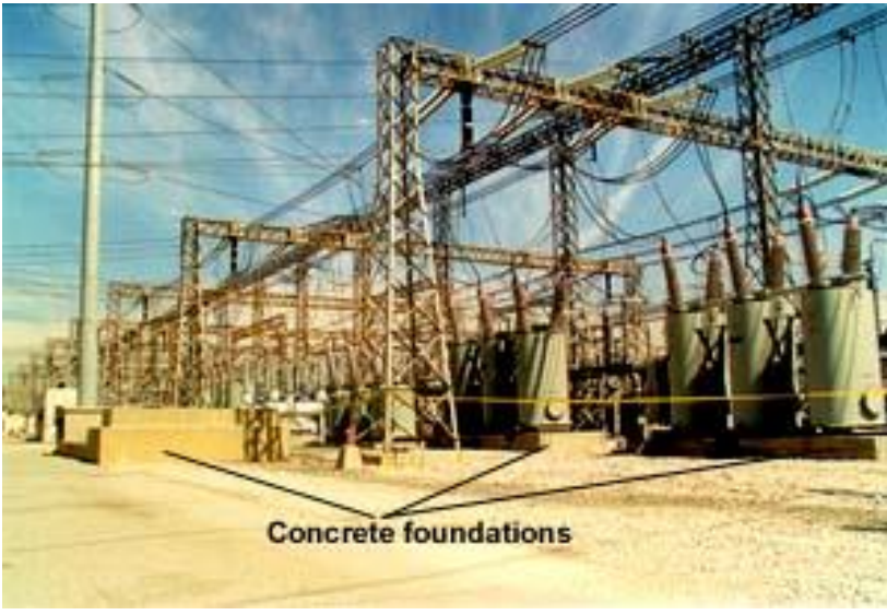
Fig: Concrete foundations
