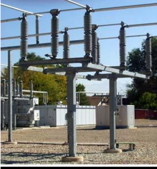
Fig: Circuit switcher
