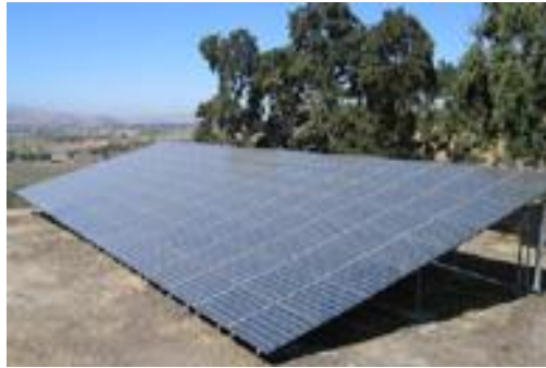
Fig 4.6: Ground Mount system.
