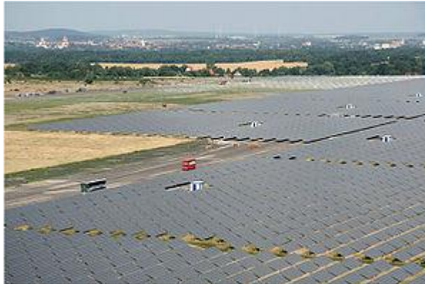
Fig 1.3: Olmedilla Photovoltaic Park[8]
