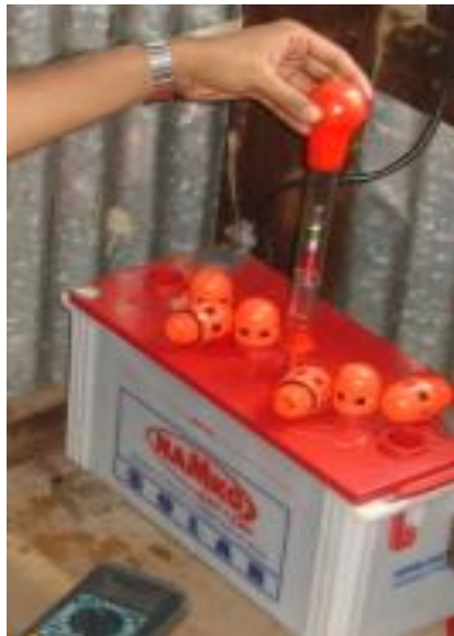
Fig 5.7: Testing of specific gravity of electrolyte of the battery cells
