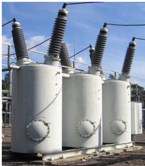
Figure: Bulk oil Circuit Breaker
