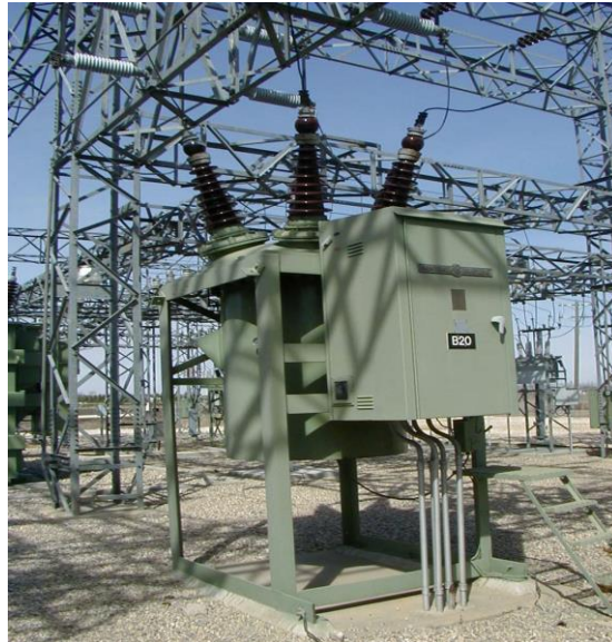
Figure: Minimum Oil Circuit Breaker
