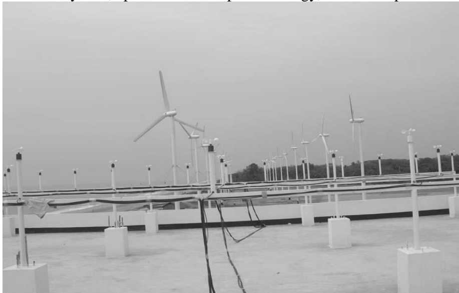
Fig: 1.4 Wind Turbines of 1000 kWp Capacity Wind Battery Hybrid Power Project at Kutubdia Island, Cox's Bazar District ( Bay of Bengal)
