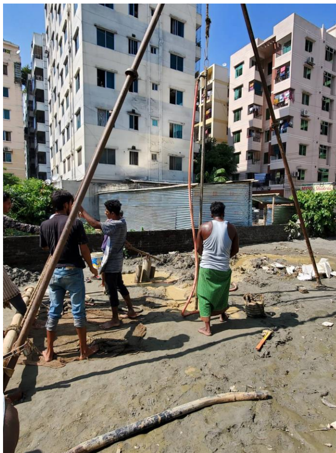
Picture 2: Standard Penetration Test (Wash Boring Method)
