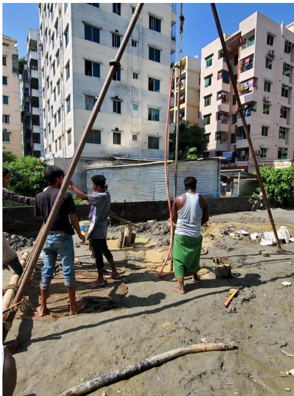
Picture 1: Wash boring
