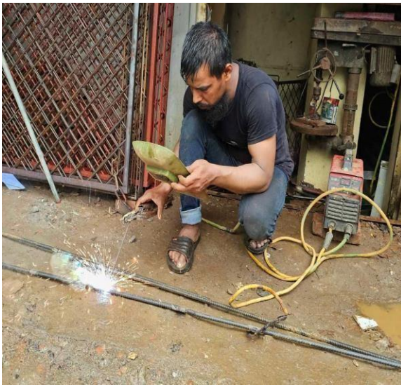
Figure 3.11: Processing of Welding
