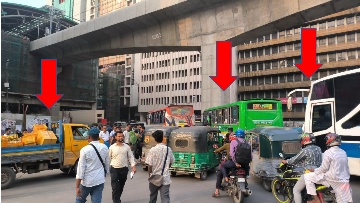
Fig 4.2 Traffic congestion at Kawran Bazar Mor. (At 8:30 am)
