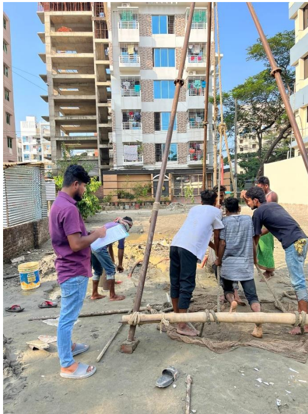
Picture 1: Wash boring
