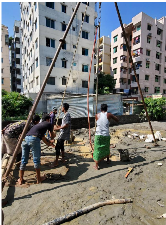
Picture 2: Standard Penetration Test (Wash Boring Method)
