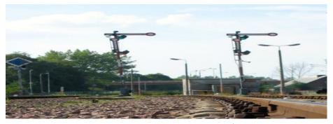
Photo 5.1: Mechanical semaphore signals at Kościerzyna in Poland
