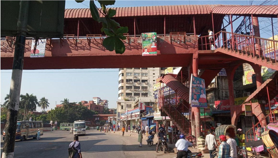
4.3.9: Footover Bridge at Farmgate.
