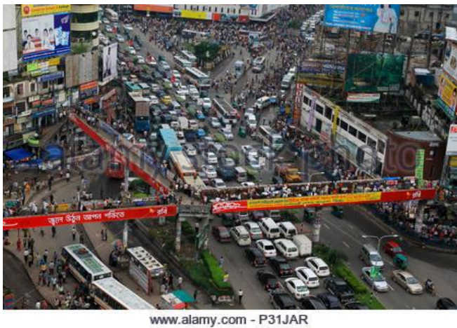
Figure 2.4.3: Foot over bridge of Farmgate.
