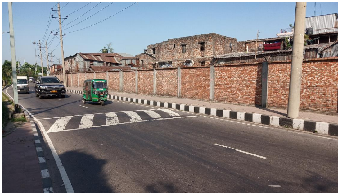
Figure 4.3.2: Narrow footpath for pedestrian which need to be widen.
