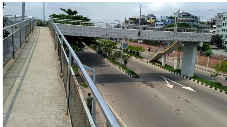
Figure 2.4.4: Foot over bridge at Hatir-Jheel.
