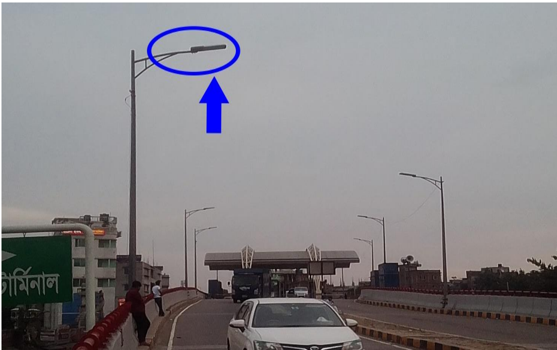
Photo 4.27: Lighting signal at Jatrabari Mayor MohammadHanif flyover
