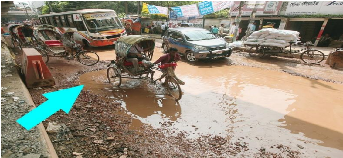
Photo 4.19: Damage Road & Stagnant Water
