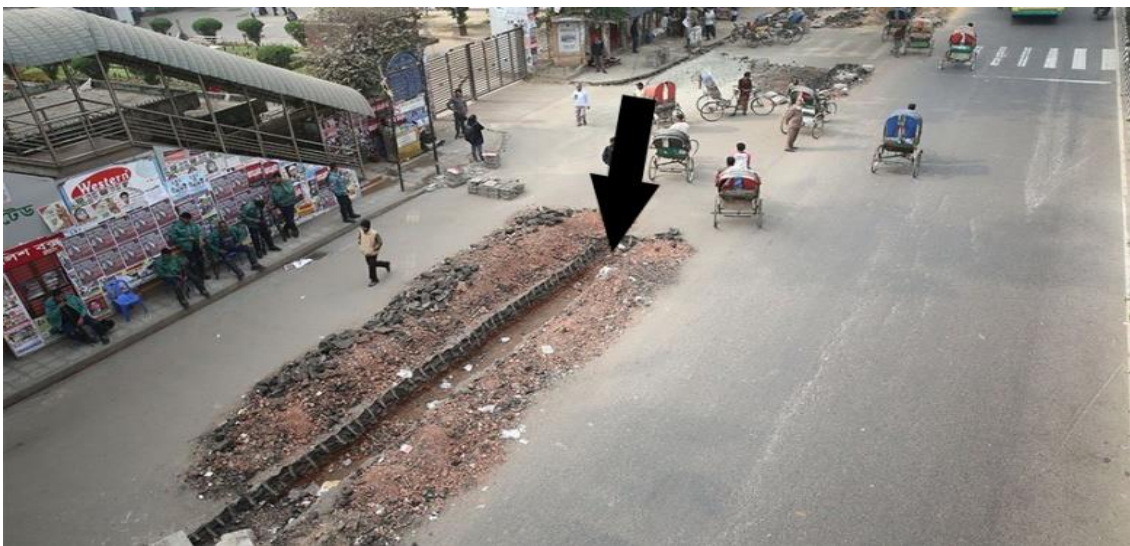
Photo 4.20: Construction Work on Road
