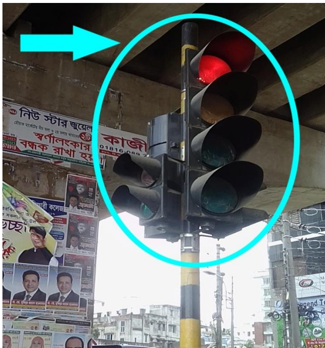
Photo 4.5: Khilgaon signal post
