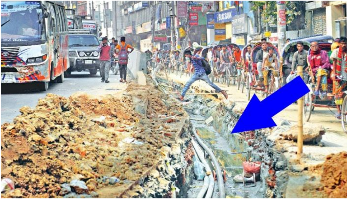
Photo 4.21: Construction Work on Road
