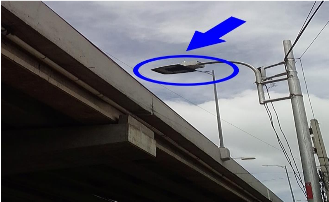
Photo 4.26: Lighting signal at Malibag
