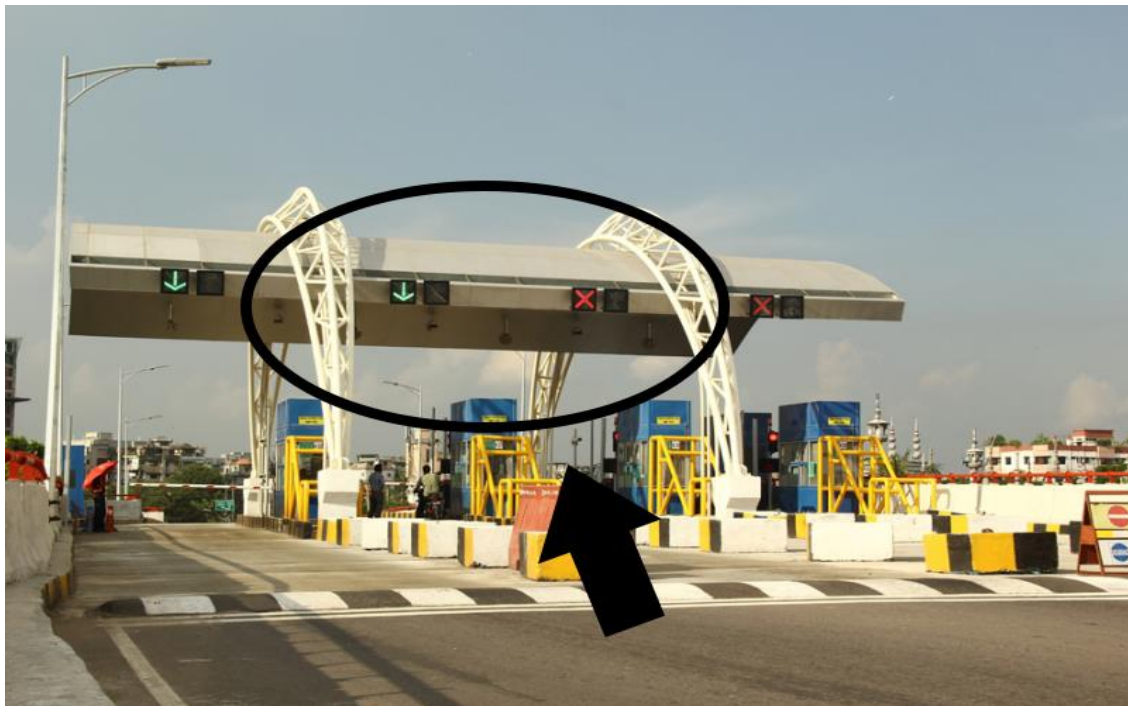
Photo 4.33: Mayor Mohammad Hanif Flyover Toll Box
