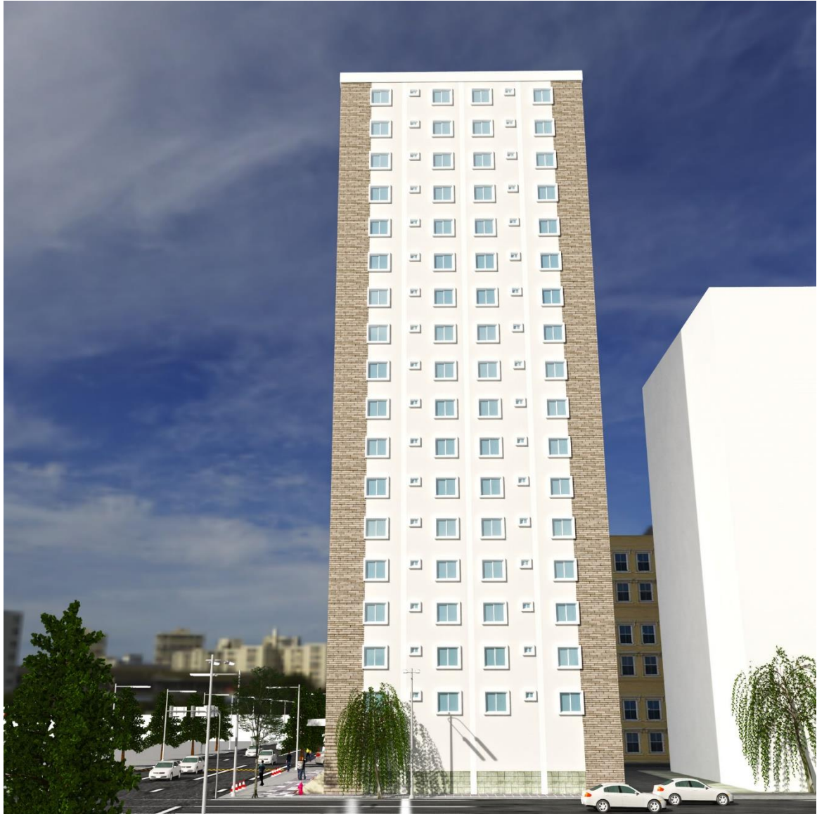
Figure 4.1c: Right side View of Building
