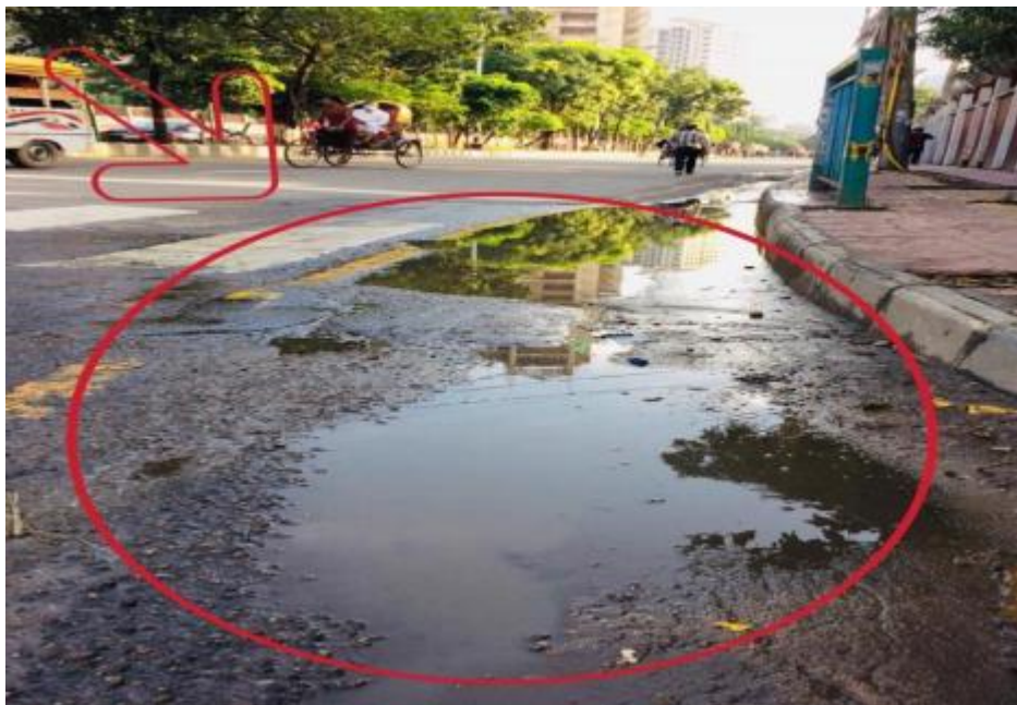
Photo 4.3: Water logged on road side of Tigerpass intersection
