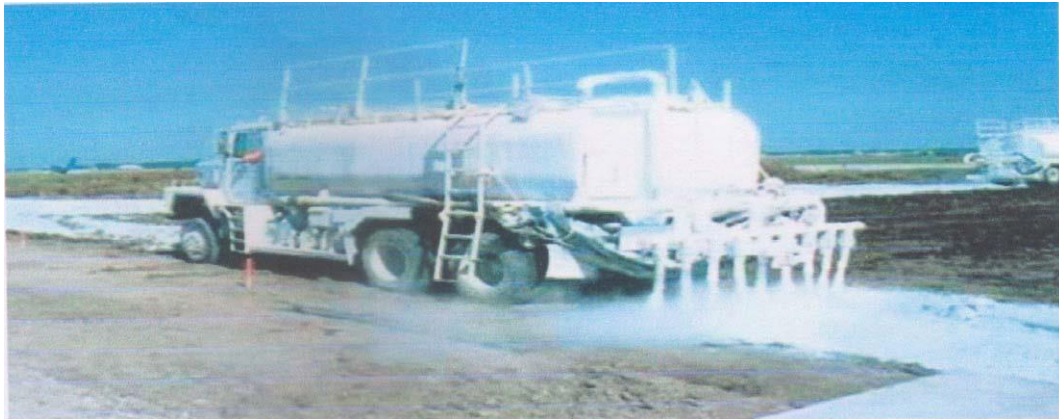
Figure 2.6: Spreading of lime over scarified soil
