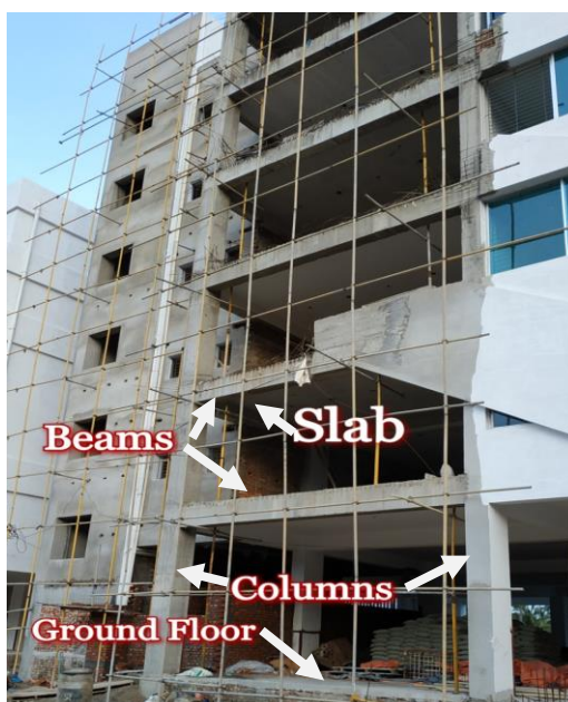
Figure 2.1: An edge supported building structure under construction
