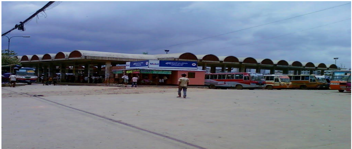
Fig 1.7: Inter-City Bus Terminal (Mahakhali)
