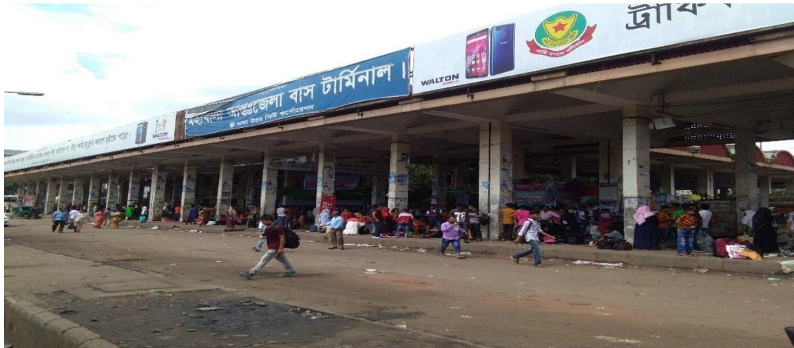
Fig 3.5: Mahakhali bus terminal
