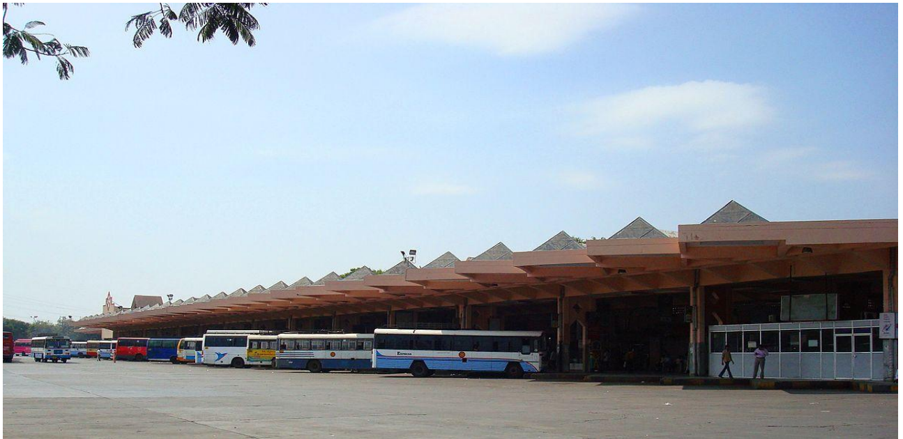
Fig 2.6: Mahatma Gandhi Bus Terminal, Hyderabad
