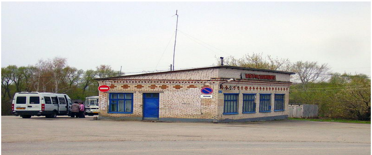
Fig 2.7: Bus station in rural Russia
