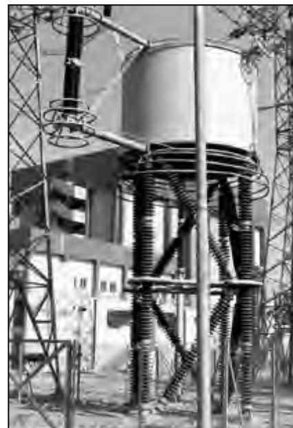
FIGURE 24.8 Installation of an air-cooled smoothing reactor.
