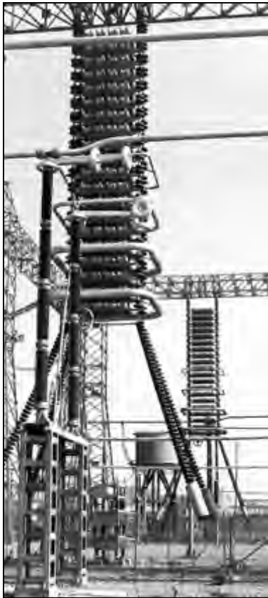
FIGURE 24.7 Installation of an ac filter in the switchyard.
